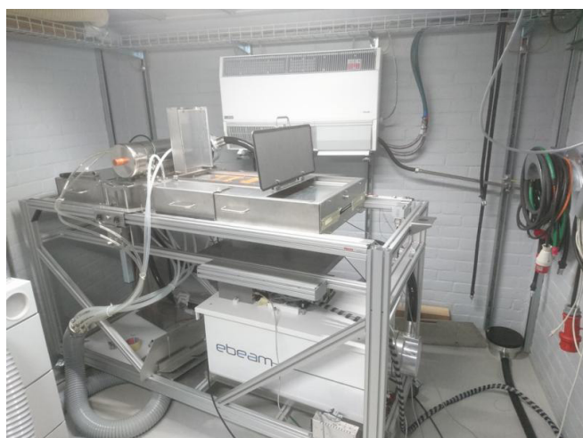
Installation ebeamTechnologies (Courtesy ebeam Technologies)
