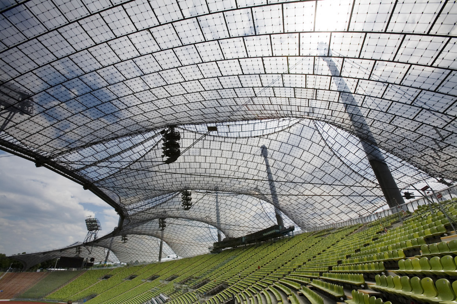
Frei Otto Olympic Stadium Park, Munchen
