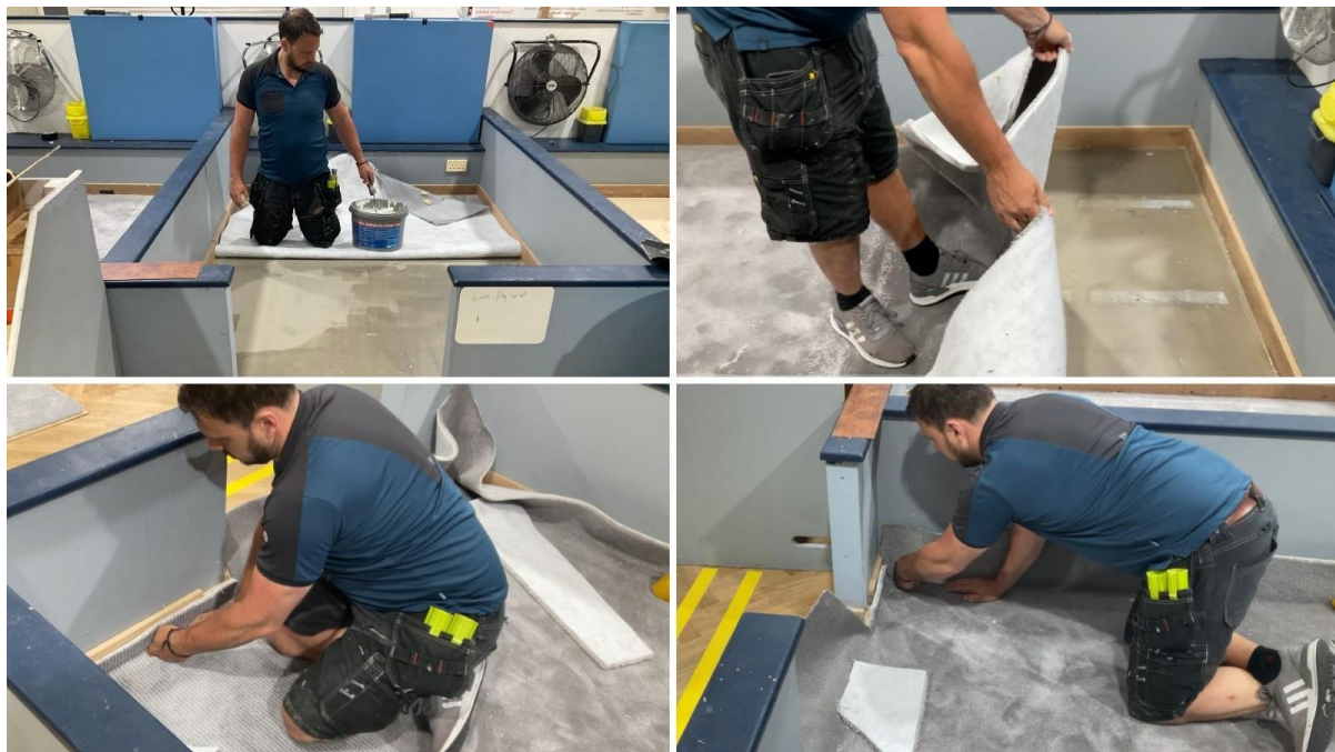
Figure 17: Stage 1 cTextile installation trials
